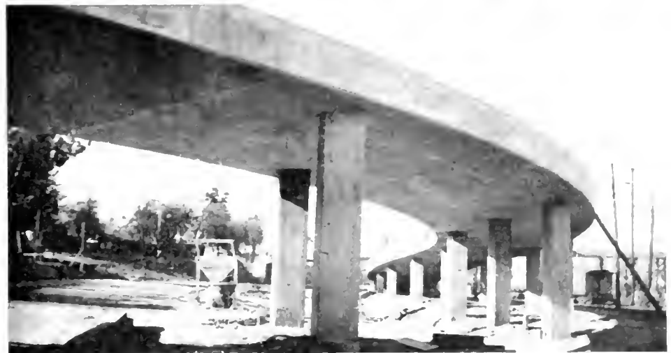
Pomeroy Street overhead, a companion traffic interchange structure to Soto Street, shows a twisting reverse curve alignment
